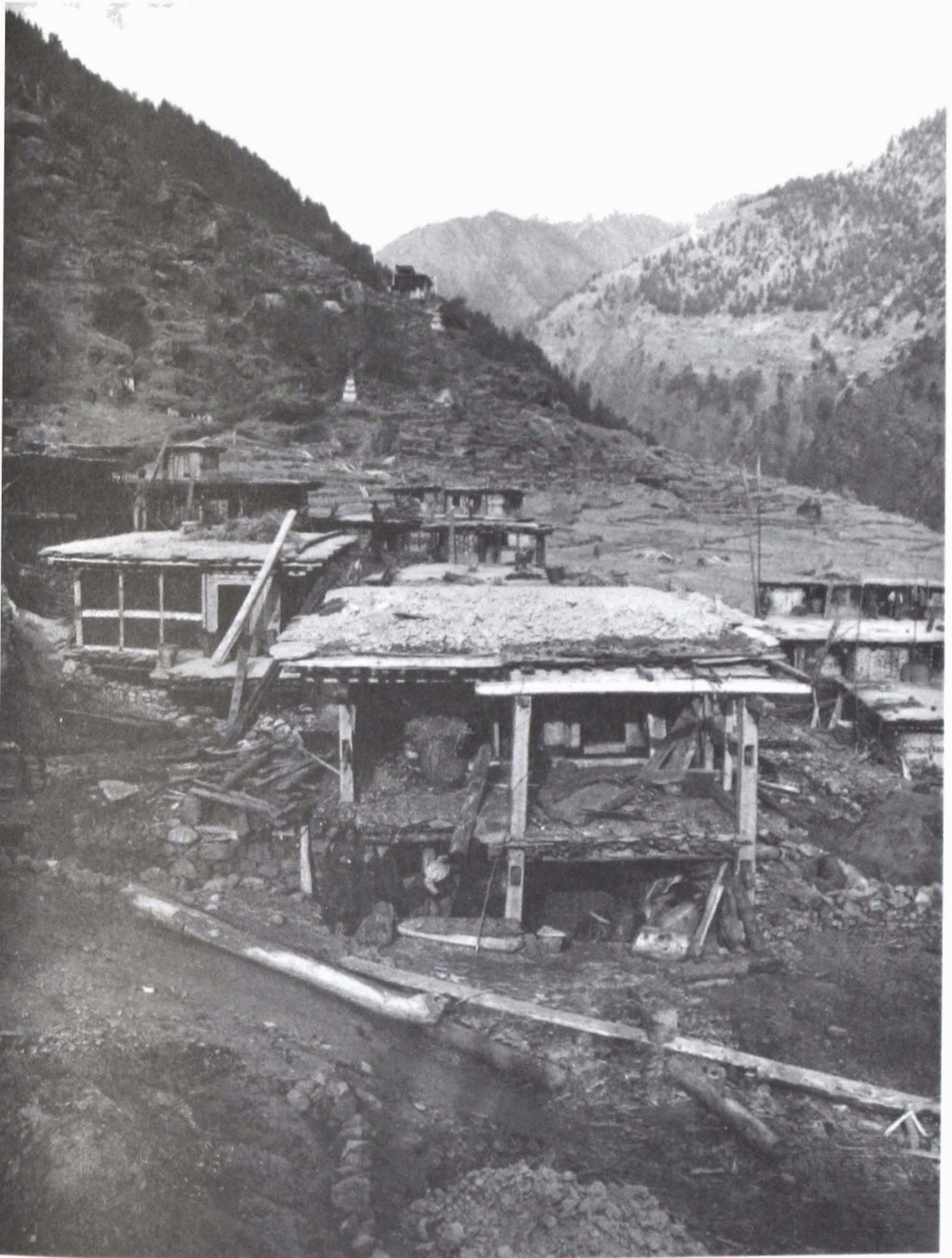
Fig. 46. A fire-damaged portion of Mangri, a Bhotia village in upper Mugu (economic region C). Construction of the homes is exposed by the various stages of repair. Note the Buddhist chortens and ghompa (temple) on the hillside beyond.
