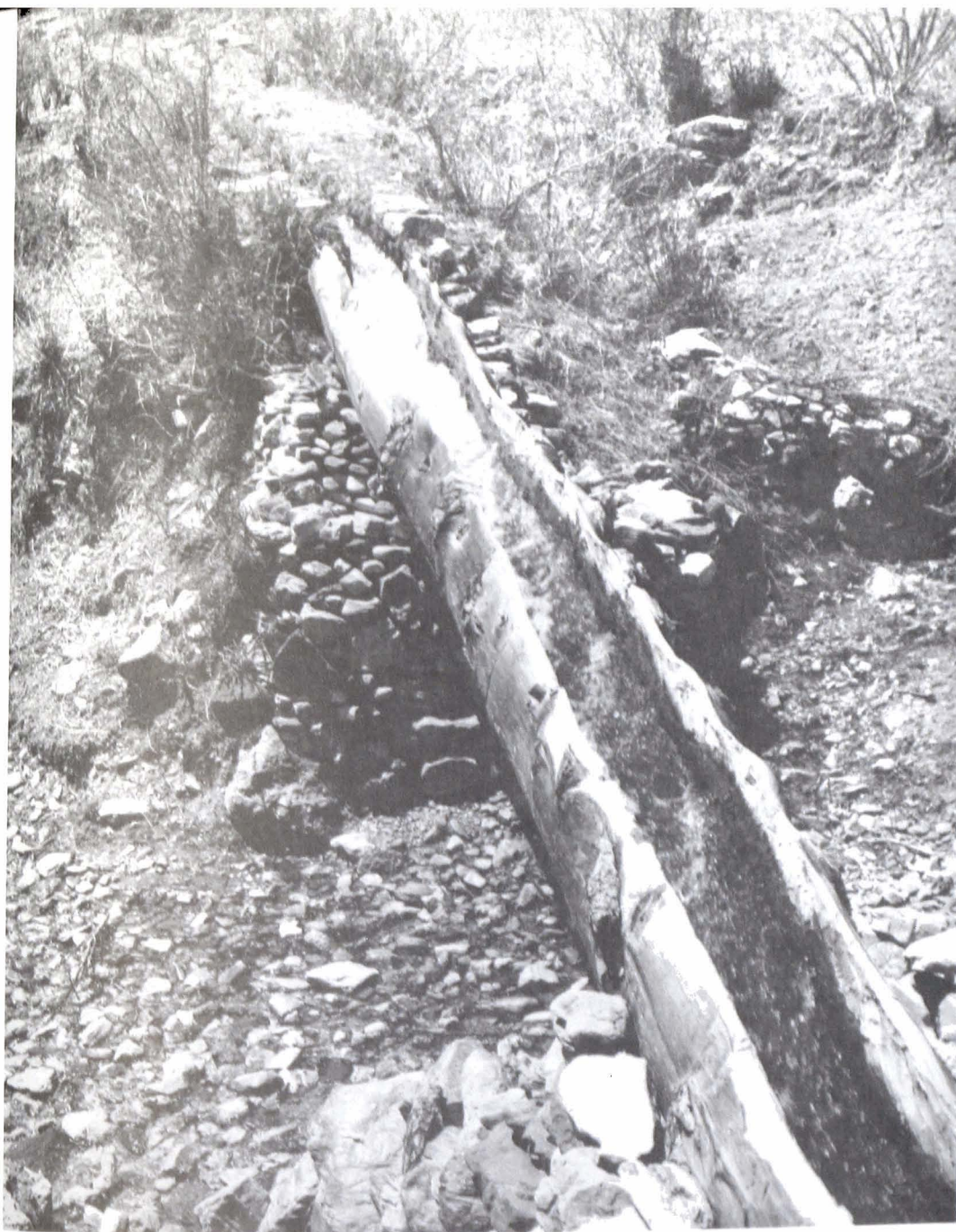
Fig. 56. A log aqueduct bridging a defile conducts water from a tributary stream to khet plots.
