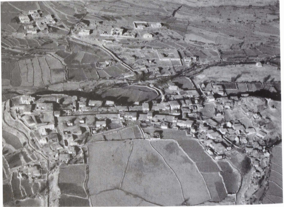
Fig. 88. December aerial view of Jumla-Kalanga looking west. Shops of the old bazaar flank the plaza in the middle ground, which is oriented north-south. Partially completed buildings of the new bazaar, where three of the zonal capital's twenty-nine shops are now located, are in the left background.
